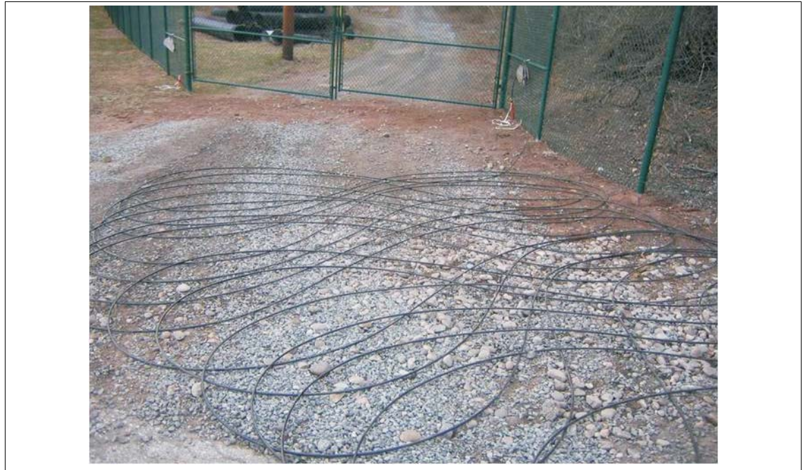
Figure 48 Laying cable in a figure-8 pattern
