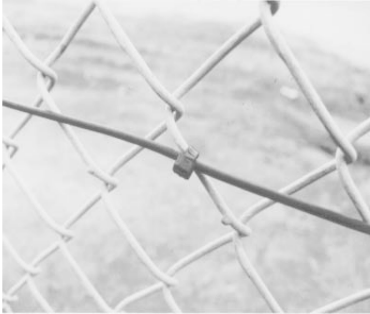
Figure 27. Cable Tie Installation
