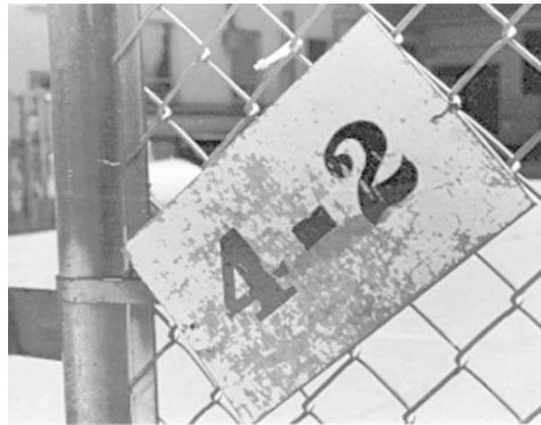
Figure 22 Signs and/or foreign objects not securely attached to the fence fabric or posts
