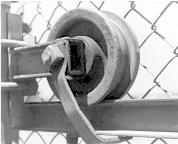
Figure 21 Too much play between rollers and rails
