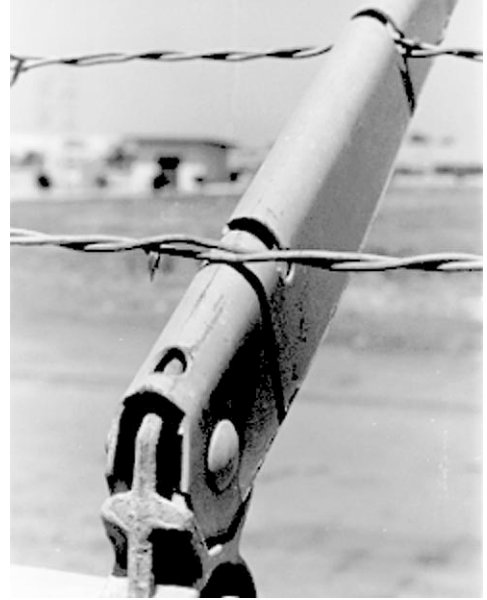
Figure 16 Barbed wire dangling due to missing keepers
