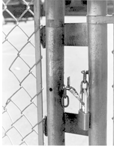
Figure 20 Chain and lock free to vibrate against gate
