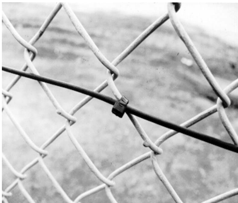
Figure 26. Cable Tie Installation
