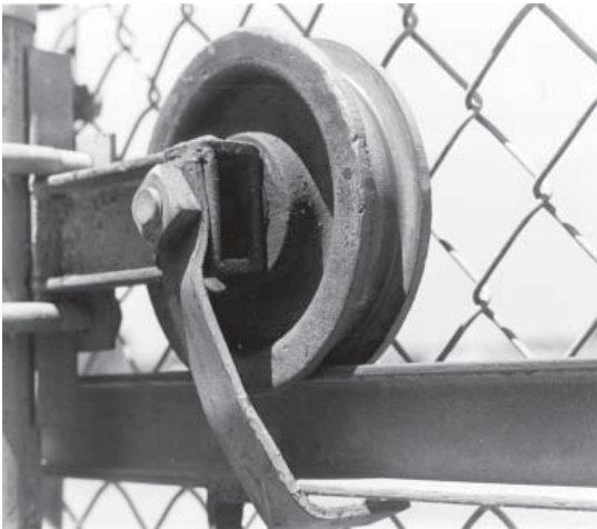
Figure 20 Too much play between rollers and rails
