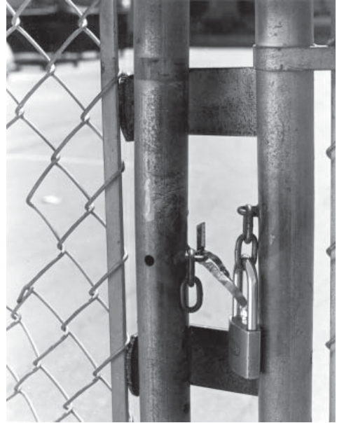
Figure 19 Chain and lock free to vibrate against gate
