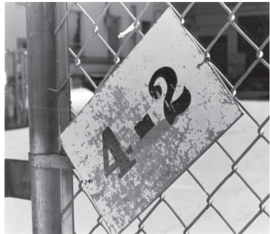
Figure 21 Signs and/or foreign objects not securely attached to the fence fabric or posts
