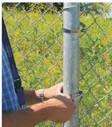
Figure 57: Post-mounting the enclosure (on the fence)
