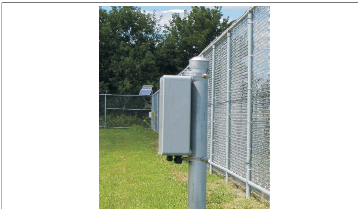
Figure 58: Post-mounting the enclosure (away from the fence)
