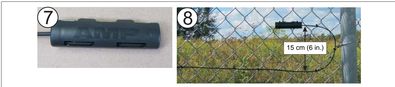
Figure 28: Mounting the termination enclosure
